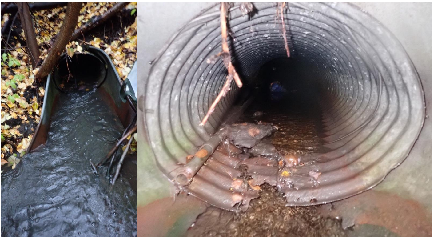
Photograph 4. Outfall SWM06 (314-22), Maplewood Street off of Northern Lights Boulevard.
