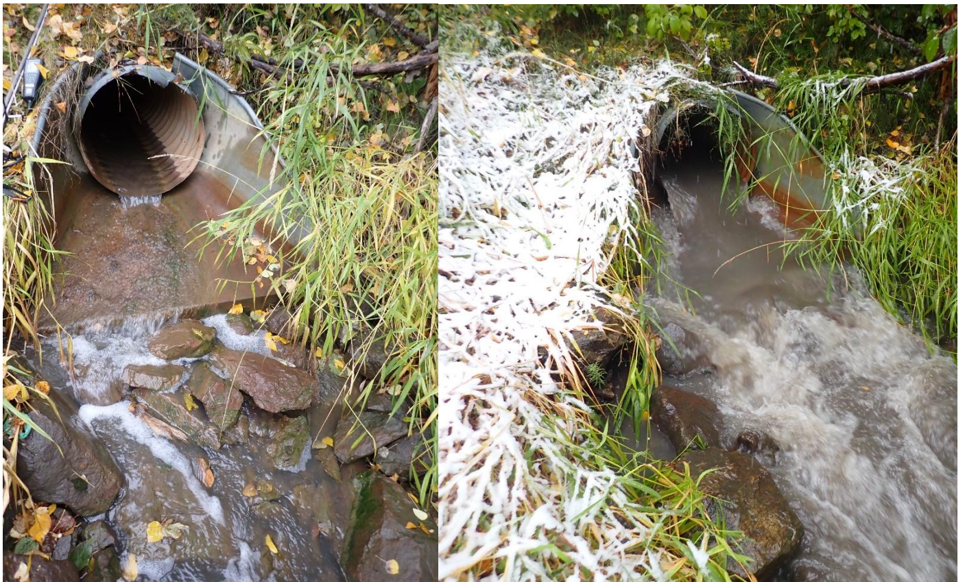
Photograph 10. Outfall SWM12 (1454-1), Lynwood Retention Basin.
