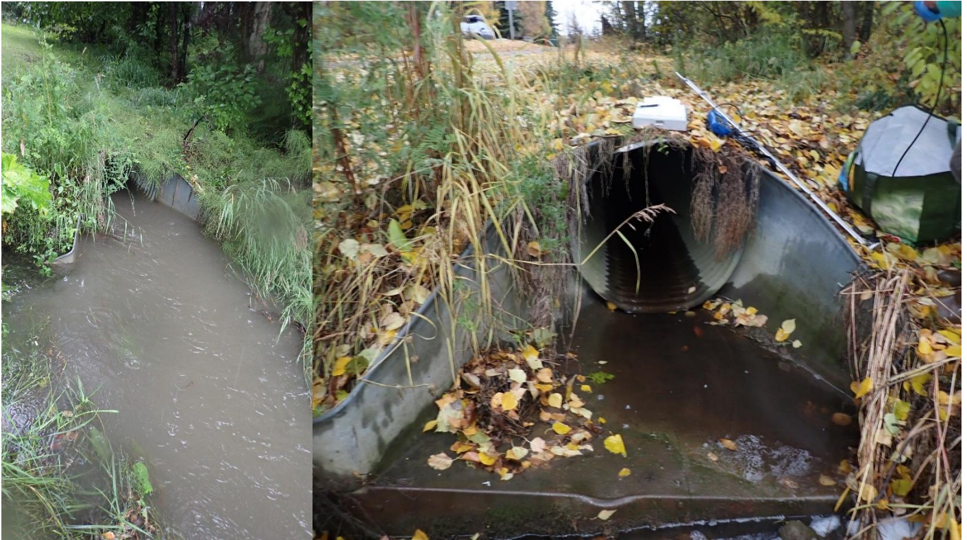
Photograph 3. Outfall SWM05 (207-1), East 56 th Avenue at Save School.
