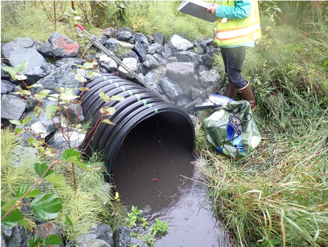
Photograph 9. Outfall SWM11 (348-3), Johns Road at Botanical Circle.
