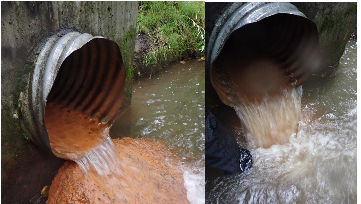
Photograph 8. Outfall SWM10 (525-2), Eagle Street at Chester Creek.
